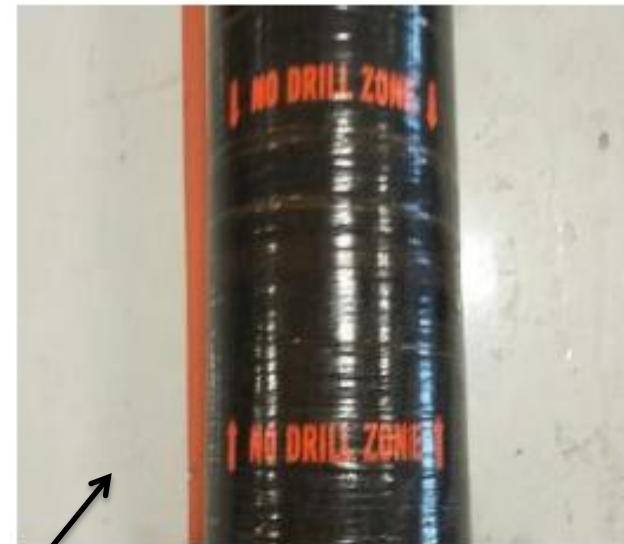
Figure 6-6. No Drill Zone Details & Markings Applied to Joint Areas
