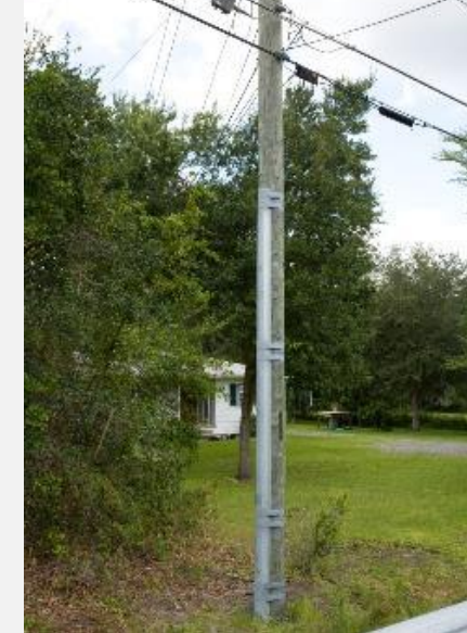
Tough Truss ® Upgrade
